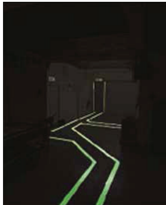
Figure 55: A 'way-guidance' system
