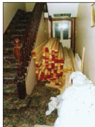
Figure 9: A blocked corridor with incorrect signage
